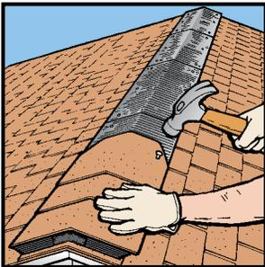
4. Center shingle cap on vent and nail. Nail line for cap shingles is to be 2"-2 1/2" up from edge. Continue nailing until all vent is covered with ridge caps. Be careful not to overdrive nail. Nail head should be flush with top of shingle, without indenting it. Pre-forming caps in cold weather helps avoid cracking.
