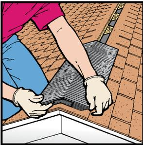
2. Nail one shingle cap at each end of the ridge, as with conventional application. Use End Plug in the exposed end on first and last sections of V-600, caulk in place. Center first piece on ridge and nail, keeping end of vent 1/2" from end of roof. Set 4 nails 1/2" from ends and 2" up from edge on each corner of vent, add 2 nails in center of vent 2" up from edge. Repeat this step at the other end of the ridge. For V-300, use the Folded End Cap technique (see Cor-A-Vent website).
