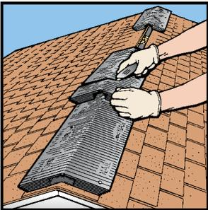
3. Continue applying COR-A-VENT, **working from ends to middle.** This technique helps remove any dips or sag at the ridge. Align center with previous piece, making sure vent matches roof pitch before nailing locator points. Continue nailing until entire ridge is covered. Use a utility knife to cut last piece to length. Caulk where bottom edge of End Plug rests on roof.
