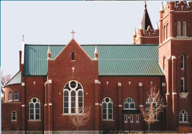
Standing Seam— All Spec Metal Systems – Holts Summit, MO
