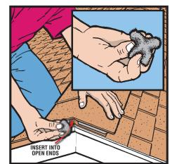
**7.** To close off ends of vent, fold over a section of End Plug material (2 per ctn.) and pinch together (see inset). Insert End Plug material between vent legs. Once seated properly, seal in place with flexible caulk.
